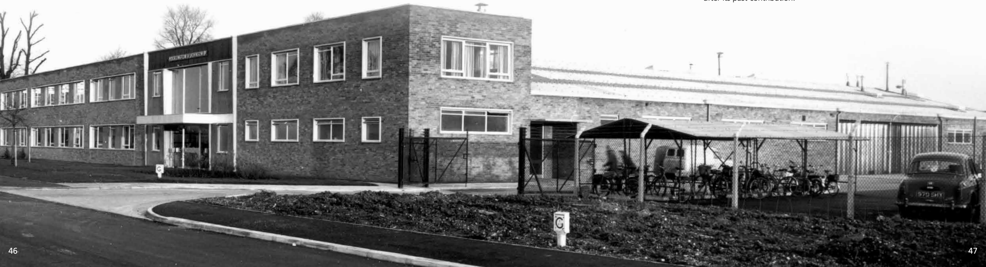
The new Watchmead premises, completed in 1971
