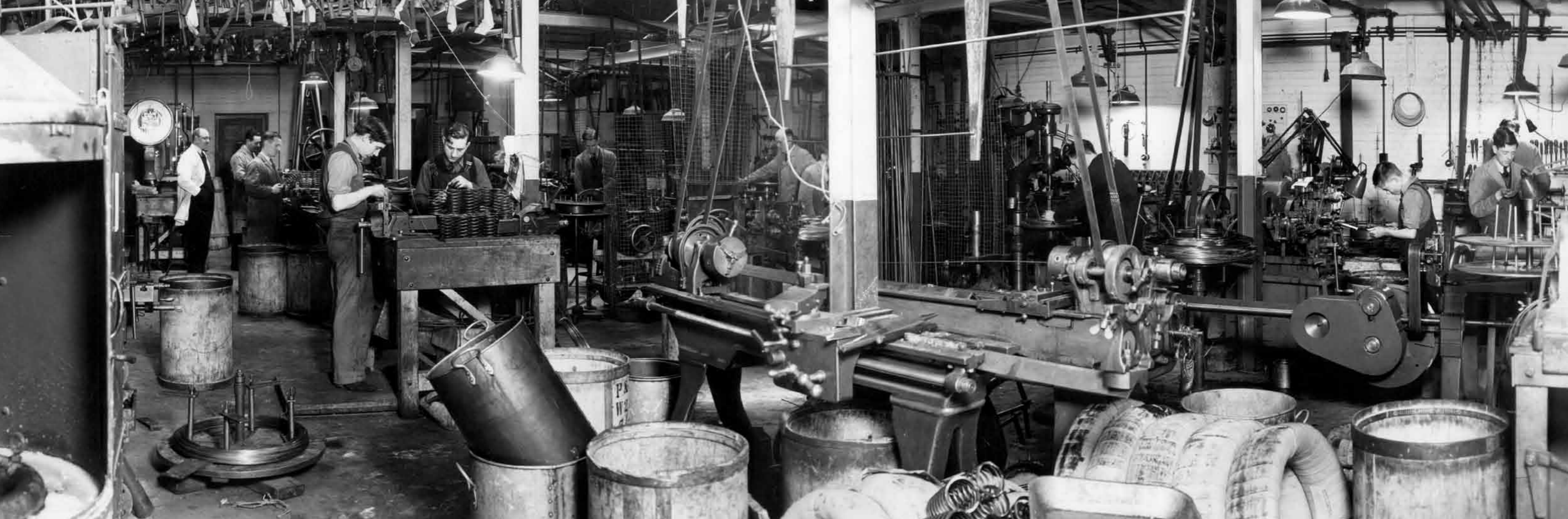
My father (far left) watches me at work at 74 Bridge Road East, early 1950s.
